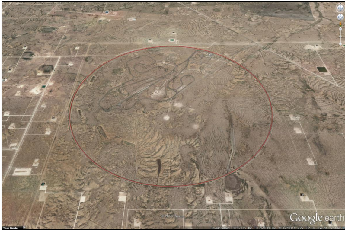
Figure 21: Pecos Test Track
